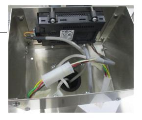
Step 4 - Reconnect HMI cover and back plate on pedestal enclosure
